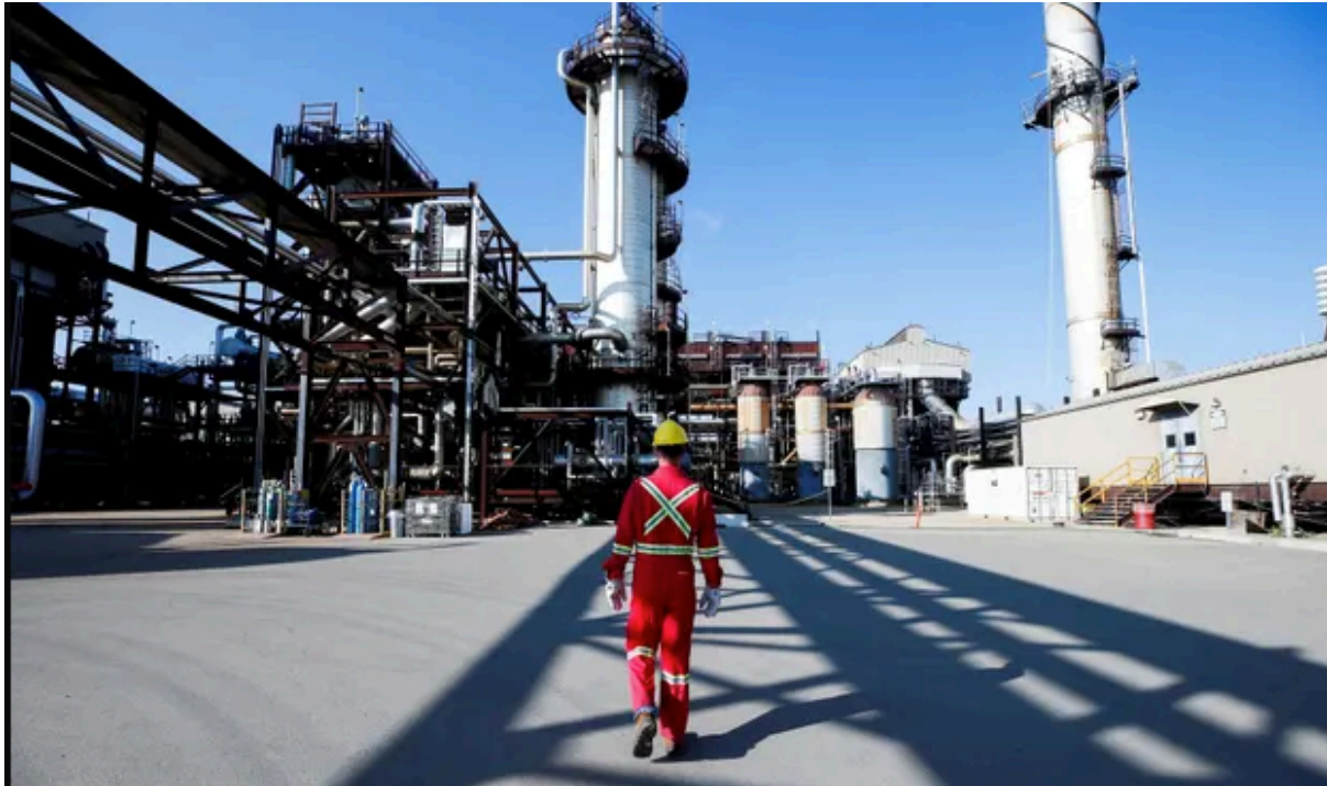
Carbon capture and storage facility in Fort Saskatchewan. Photograph: Todd Korol/Reuters
